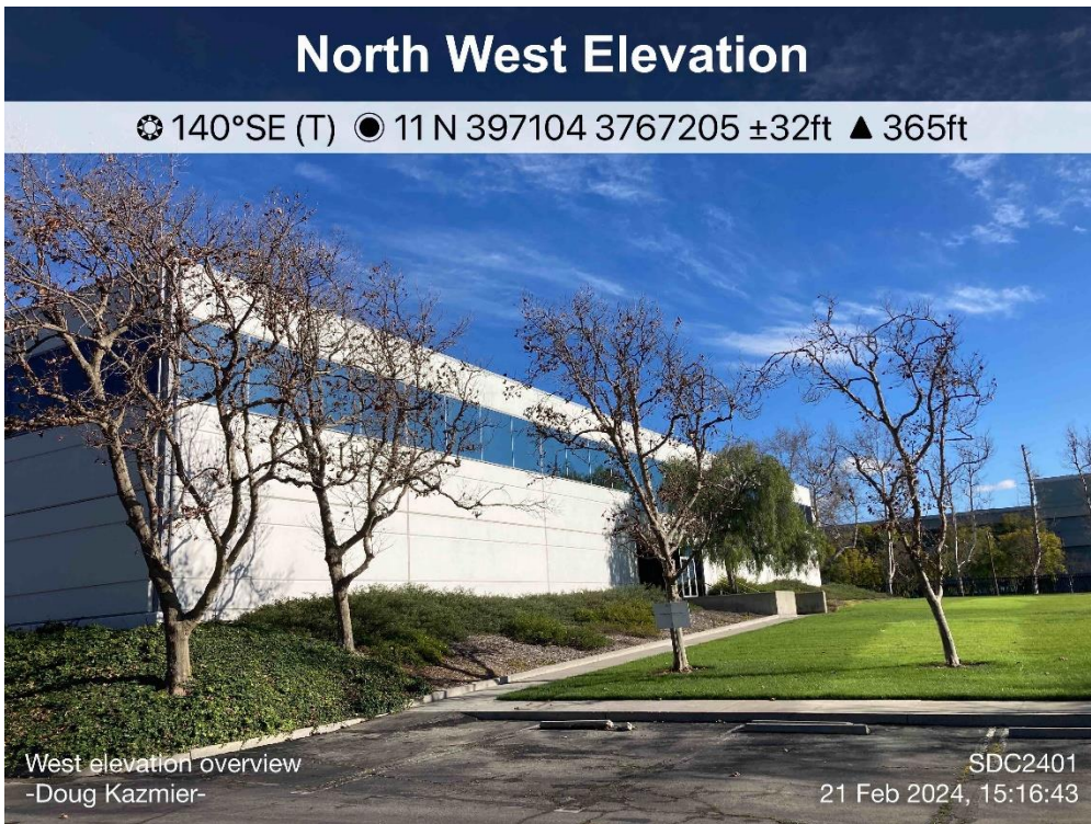
Photo 6: Overview of NW Corner of Building
