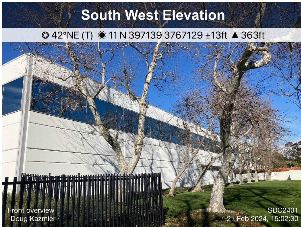
Photo 2: Overview of SW Corner of Building
