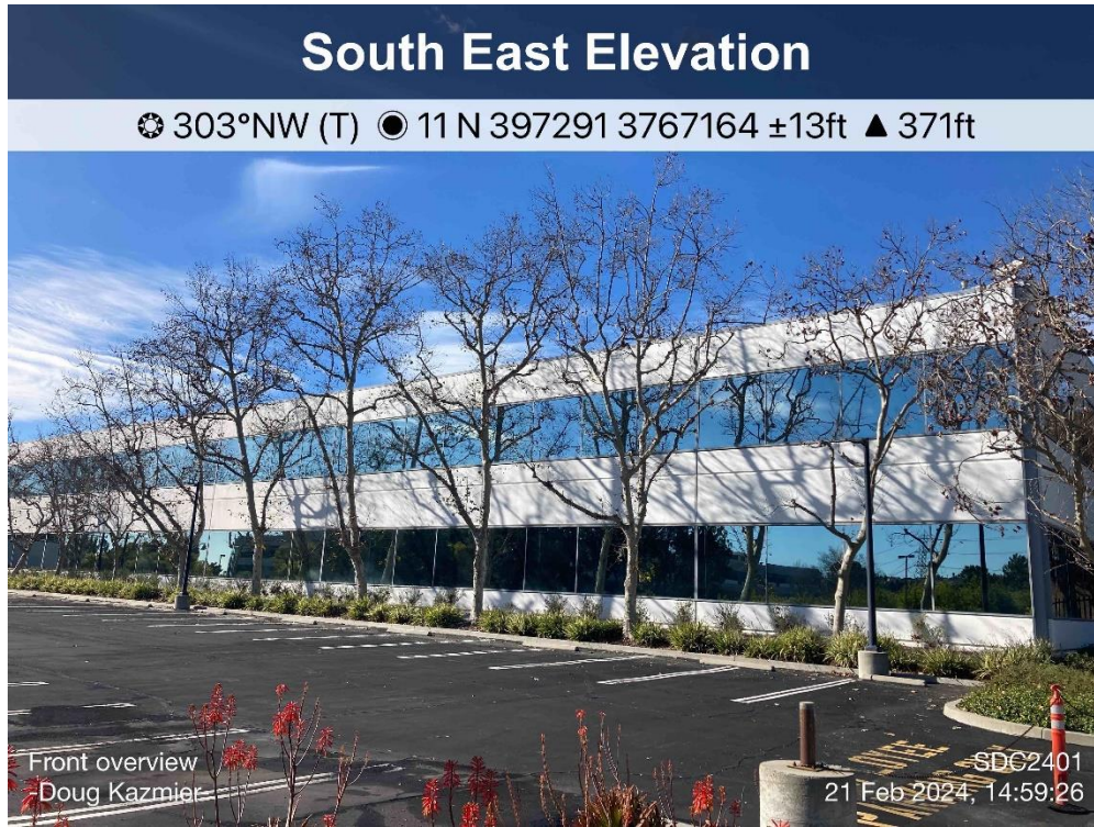
Photo 1: Overview of SE Corner of Building
