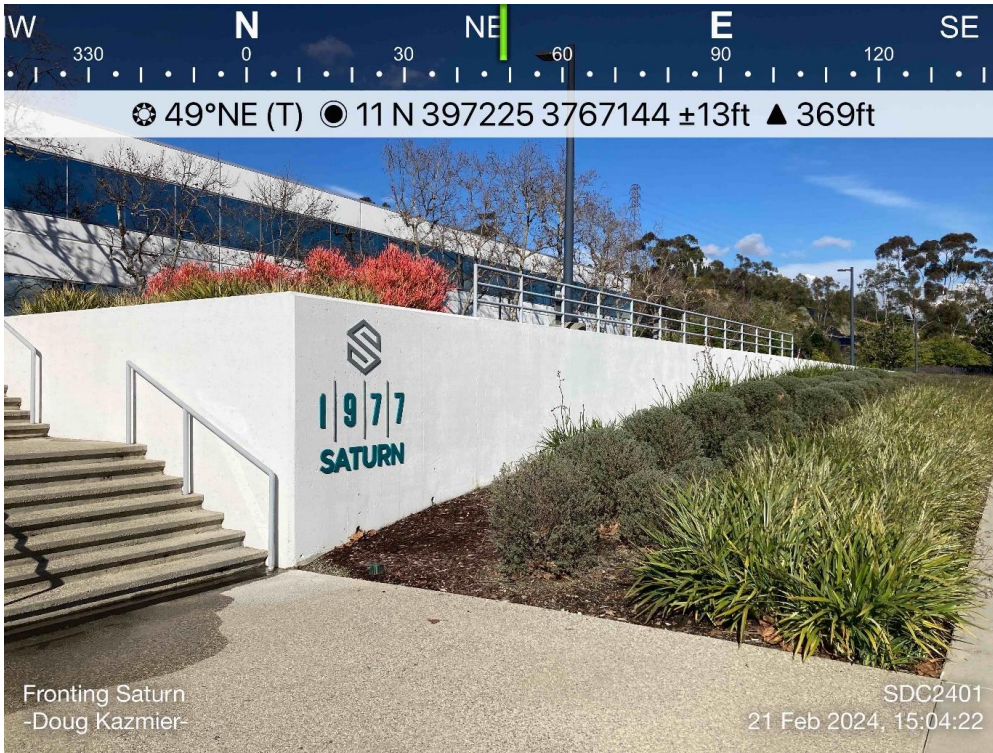
Photo 3: Overview of Building Entrance Path on S Side
