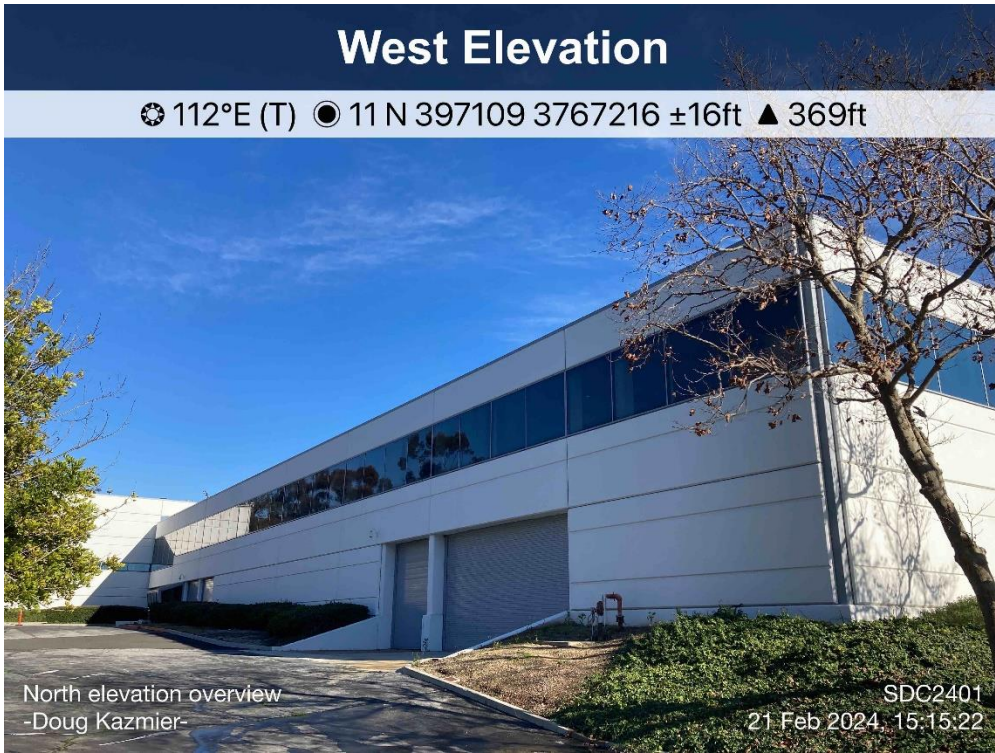
Photo 5: Overview of NW Corner of Building
